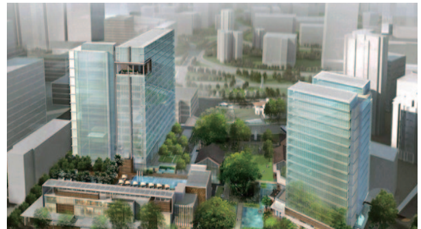
Smoke control system - Zhong Shan Park
