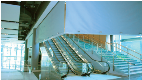
Smoke control system - Singapore Expo
