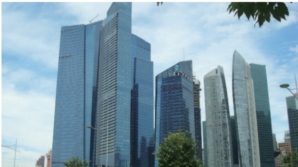
Smoke control system - Marina Bay Financial Centre
