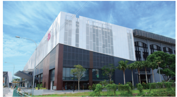
Smoke control system - Ten Mile Junction
