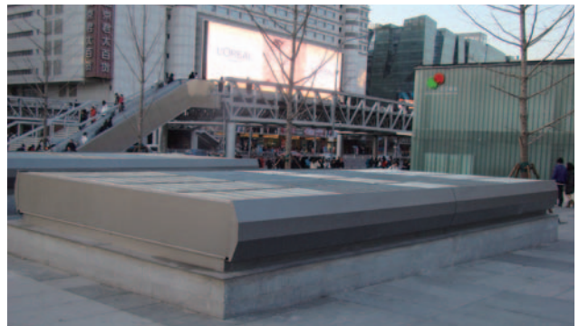
Horizontal Performance Louvres - Beijing MRT, Line 4
