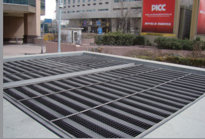
Horizontal Performance Louvres - Beijing MRT, Line 4
