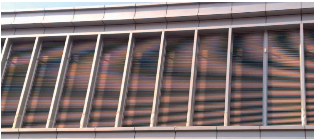
Single Bank and Double Bank Ventilation Louvres - Zhongjie Heng Lung Plaza, Shenyang
