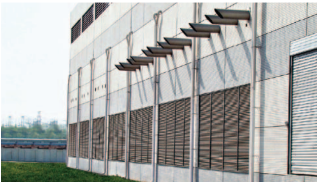
Double Bank Rainproof Ventilation Louvres - Maode Cell Plant, Chongqing
