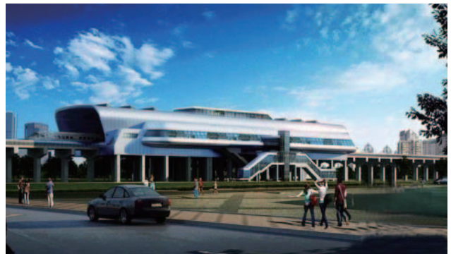
Horizontal Performance Louvres - Beijing MRT, Line 4
