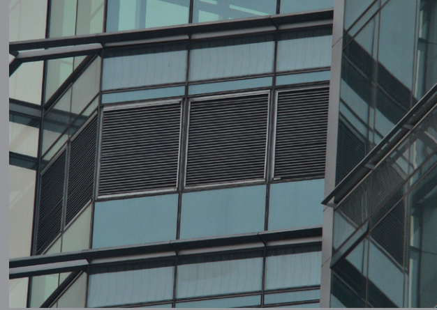
Double Bank Rainproof Ventilation Louvres - Beijing Hua Trade Centre
