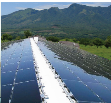
Thin Film Solar Cell Installation - Memmingen
