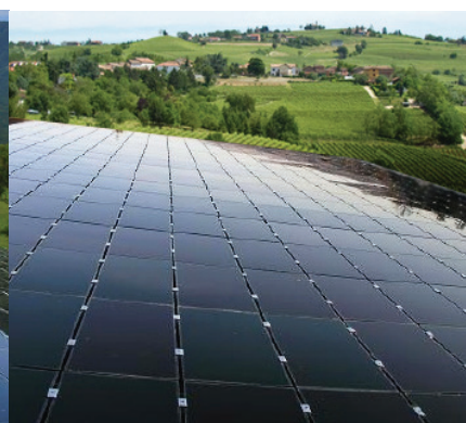
Thin Film Solar Cell Installation - Katzenbach
