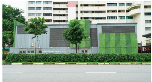
Single Bank Performance Louvres - Tampines East MRT station
