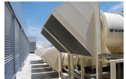
Powered Smoke Extraction Fan
