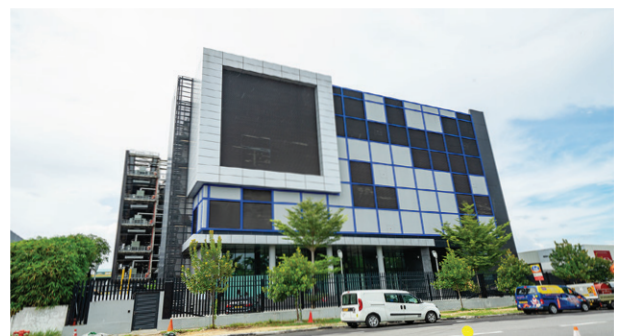
Double Bank Performance Louvres - DRT Loyang Data Centre
