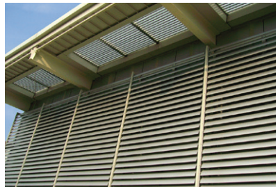
Movable Solar Shading System - Shanghai Dazhong Plant
