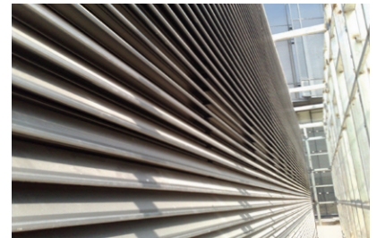
Double Bank Performance Louvre (DBL) System - Shanghai Expo Centre
